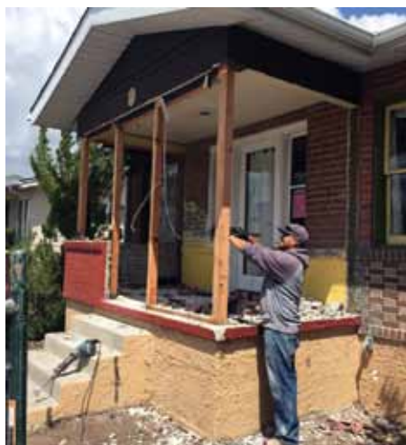
Dismantling the vestibule.
