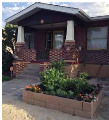
The new porch and the raised garden.
