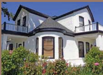
A 2016 NPF Grant helped refresh the paint on 542 Lander Street. Photo courtesy Cindy Ainsworth.
