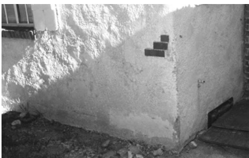
803 Nixon, before on left, after the masonry repairs on the right.
