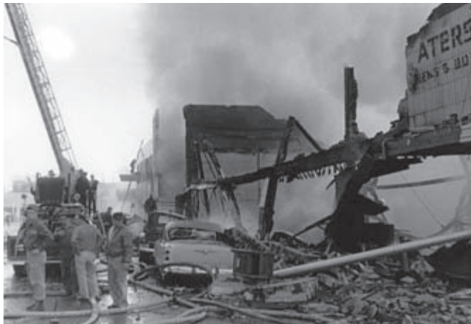
All that remains of the blast origin is twisted steel and rubble. Note the abandoned automobiles. Photo by Steve Johns.
