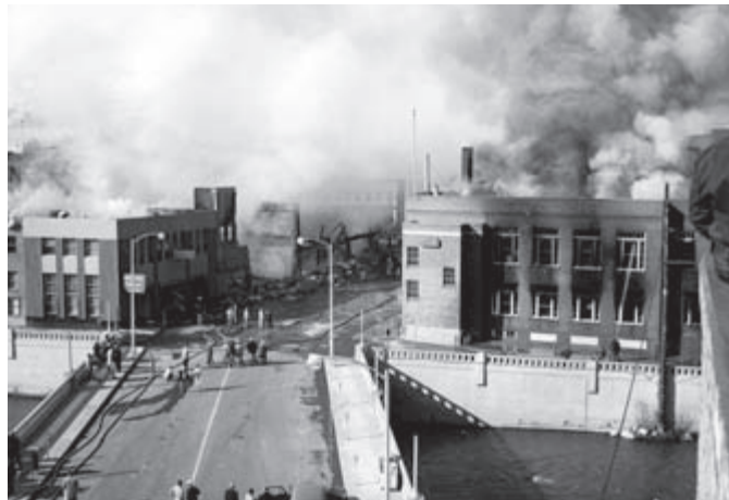
Looking north from the Sierra Street Bridge, the Elks Club burns on right and the Sanford-Biltz building burns on the left with the heart of the blast in the center of the photo.
