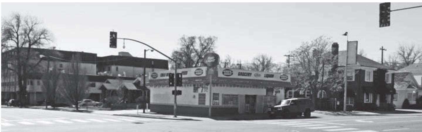
Southwest corner of Ralston and 2nd streets, where the grammar school would have been built. Photo courtesy author.
