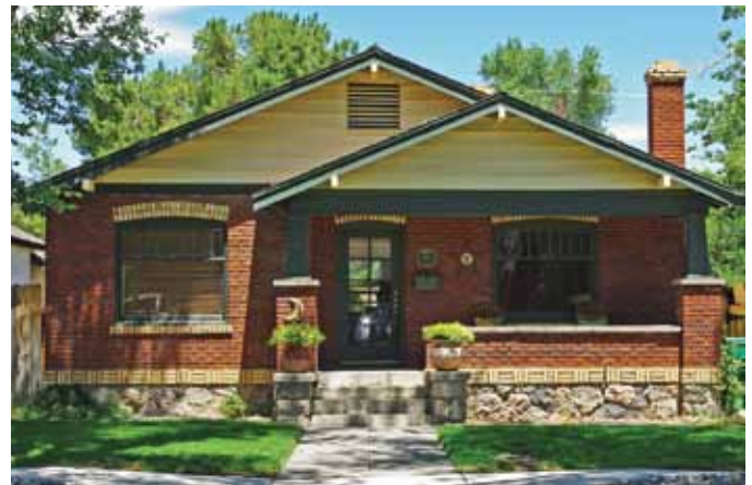
569 W Taylor: This is an example of a Craftsman bungalow with decorative brick elements. Note the red brick walls, which contrast with the light brick rowlock lintels, rowlock sills, and basket weave water table course.
