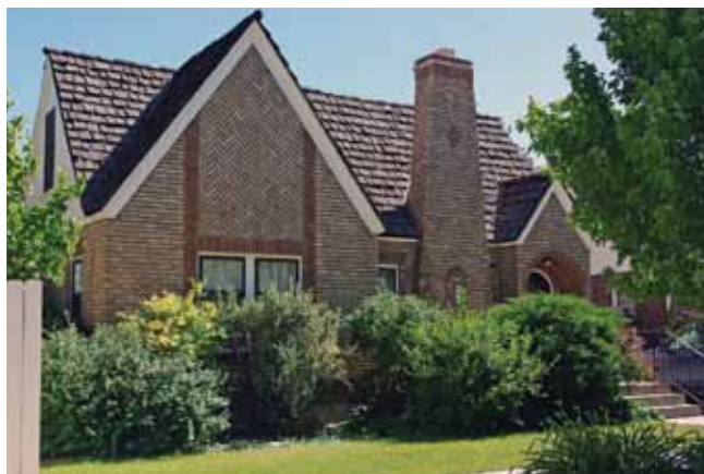
620 St. Lawrence: This Tudor Revival cottage has contrasting brick trim around the doorways, windows, and chimney cap; a diamond-pattern inlay in the chimney; and a herringbone pattern in the end gable.
