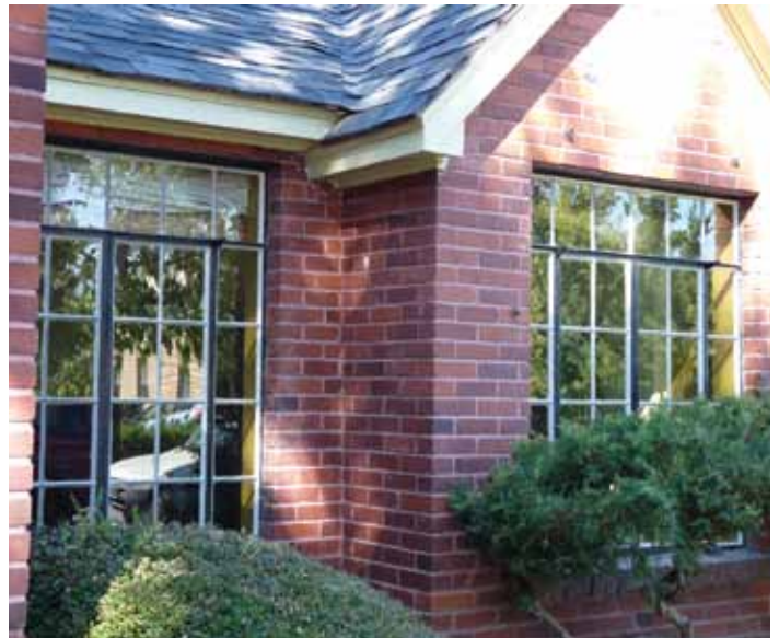
A 2014 NPF grant enabled the owners of 637 Saint Lawrence Avenue to replace 100 panes of broken, stained and poorly glazed glass while retaining the original metal windows.
