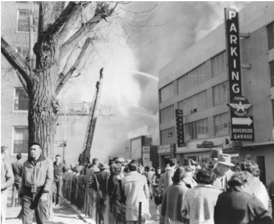
On February 5, 1957, two major explosions occurred, centered on Sierra Street between First Street and the Truckee River. Gas lines ruptured beneath the street. Tony's Deli at 150 W. First Street was impacted by a 2-week closure. Photo courtesy Neal Cobb.
